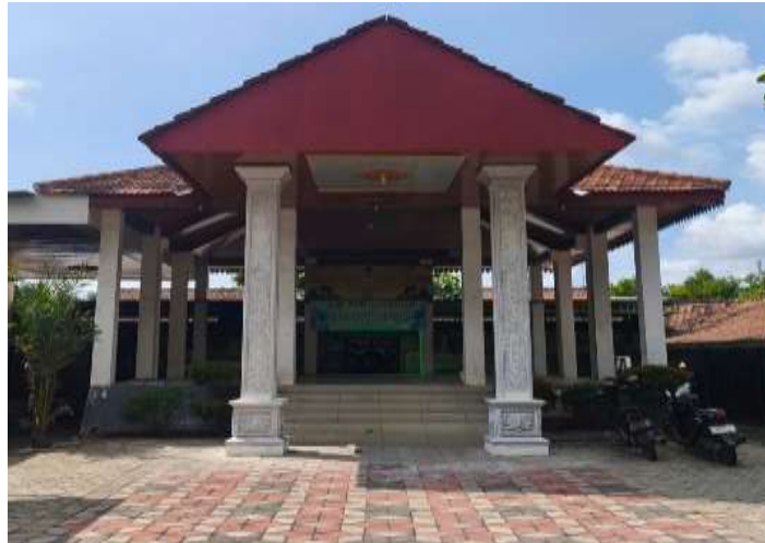
Figure 1. Results of the construction of the Karangrejo Village pavilion in 2024
