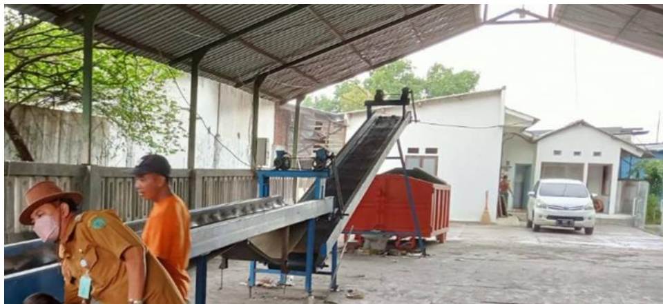
Figure 1. Condition of the roof of the Kedungturi TPST after revitalization :
